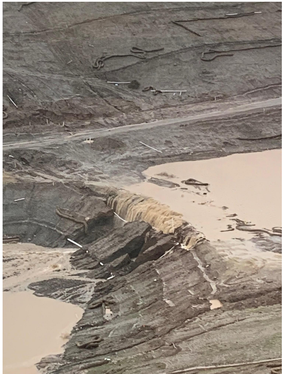
Photo 2: Looking west at the berm between Basin 8 and Basin 9, taken during the December storms. A period of intense rainfall resulted in a washout on the slope of the berm.
